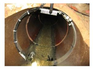
The upper sections of the collection system presented a different challenge. Shallow flows were such that the velocity and pressure sensors remain out of the flow during periods of low flow as illustrated in the picture to the left.
