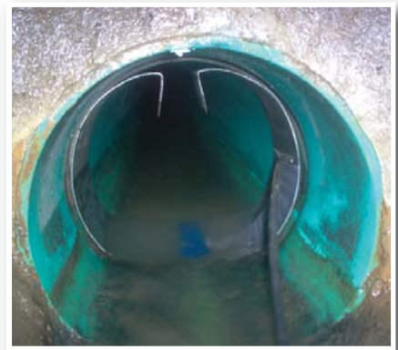
Probe and band in sewer.
