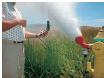
Fire Flow Testing
