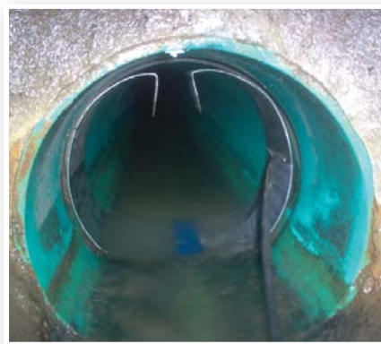
Probe and band in sewer.
