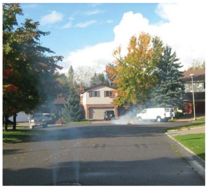
Smoke testing was carried out on roughly 20 km of sewer and service laterals of the Lo-Ellen Park area.
